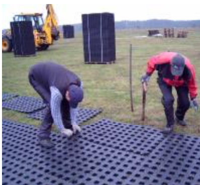
Sections arranged on the ground
