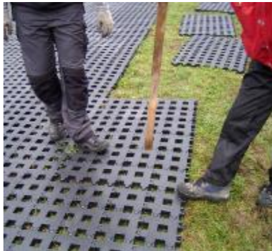
Perfo sections clipped together using foot pressure on the clips
